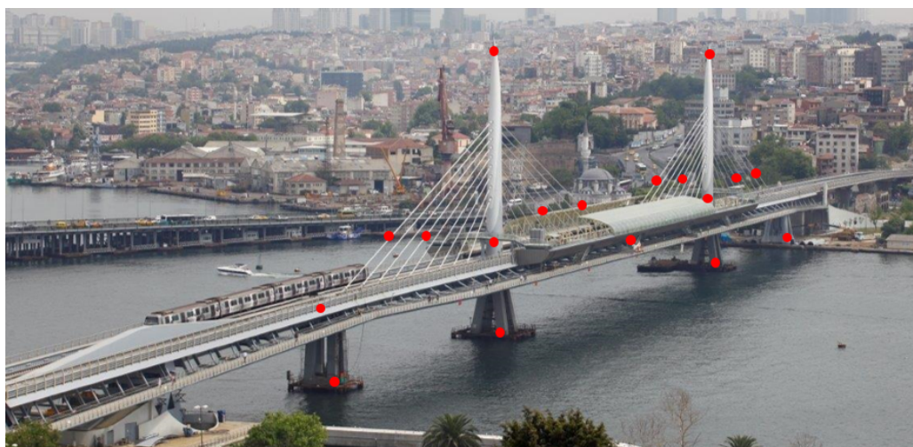
Figure 4.13 : Permanent acceleration sensors' location.
